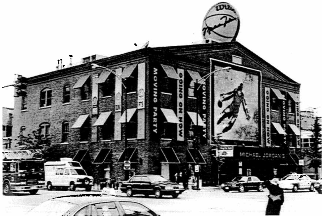
In recent years the LaSalle Cable Car Powerhouse has housed restaurants. Top: Ireland's, seen here in a 1986 photograph, was a long-popular seafood restaurant. Above: The building more recently housed a restaurant named for the NBA basketball star, Michael Jordan.
